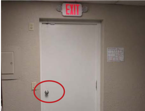
Exhibit 4-22 Northeast Exit Door with Conventional Door Knob Installed
